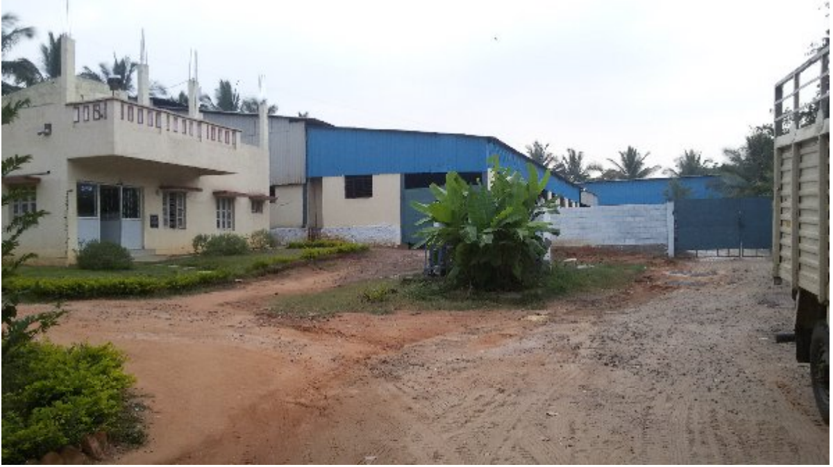
FACTORY AND ADMIN BLOCK
